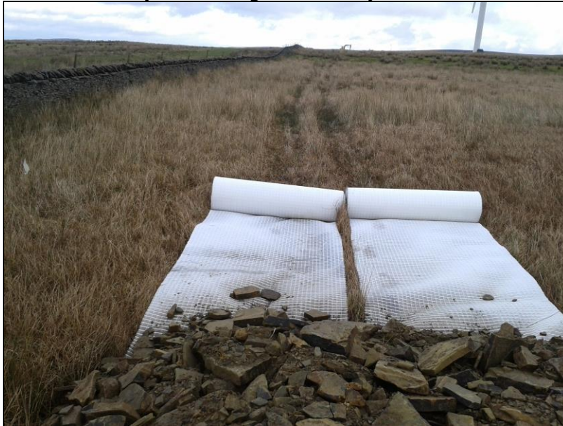
Plate 13: semi-permeable geotextile layer
