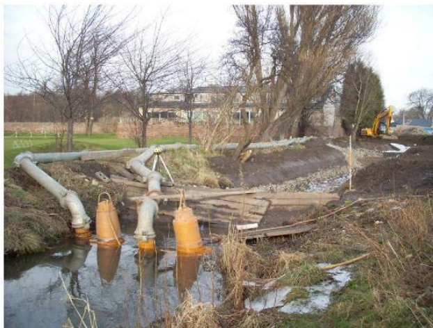
Plate 8: Full isolation – over pumping/siphon
